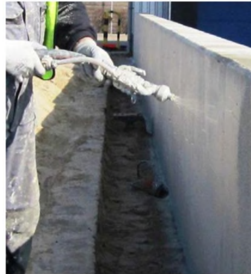
Imaginea 2: Aplicarea prin spreiere a MasterSeal 6100 FX
